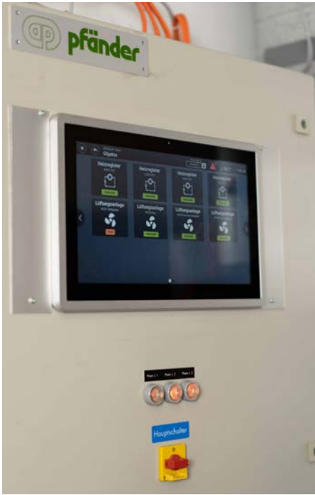
FIGURE 6a,b: The maintenance supervisor can use an operating panel to read out the data from the ventilation system at any time and adjust it manually if necessary.
